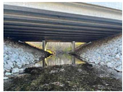
Photo 634. Prairie Creek - Looking east (upstream) along Prairie Creek and the riprap lined spill slopes under INDOT Bridges I65-142-05571 BSBL and BNBL.
