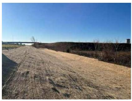
Photo 633. ROW - Looking south at erosion blanket along the roadway sideslope of the I-65 SB travel lanes associated with the I-65 ATL project.
